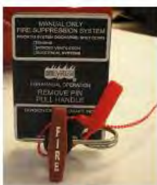
Figure 5: Pull Handle with Safety Pin and Tie
