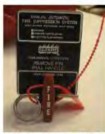
Figure 5: Pull Handle with Safety Pin and Tie
