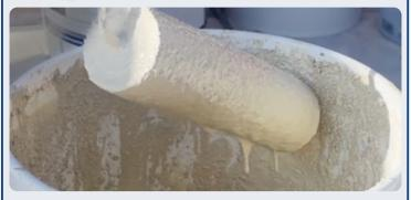
Pour Pettit Tuff Coat into a 5 gallon bucket (combine multiple gallons if possible). Lightly dampen Tuff Coat Textured Roller with water. Dip roller into the bottom of the 5 gallon bucket and spin the roller a few times, completely saturate the roller with Pettit Tuff Coat. Leave no bare spots on the roller.
