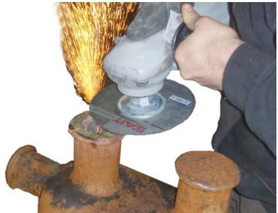
Figure 2-Grinding the Selected Horn
